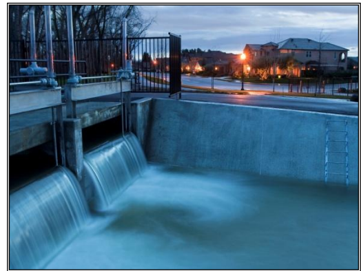
Enterprise Flume and Canal - Fresno Irrigation District
