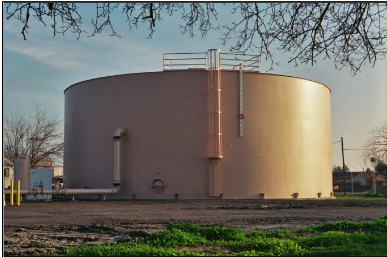
Water Storage Tank in Western Fresno County
